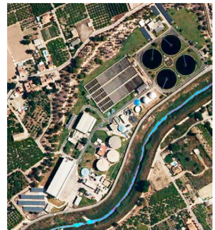
Figure 1. Orthophoto of the WWTP under study (Source: IGN's Iberpix cartographic viewer).
